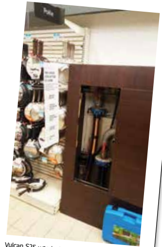
Vulcan S25 was installed in the water main to treat the whole building.
